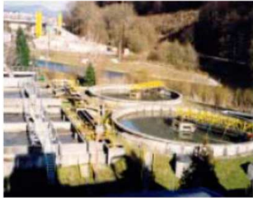
Waste Water Treatment Plant – Poland
